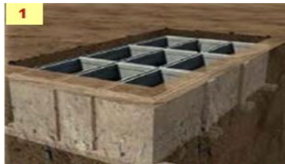
View of preinstalled CBS crypts
