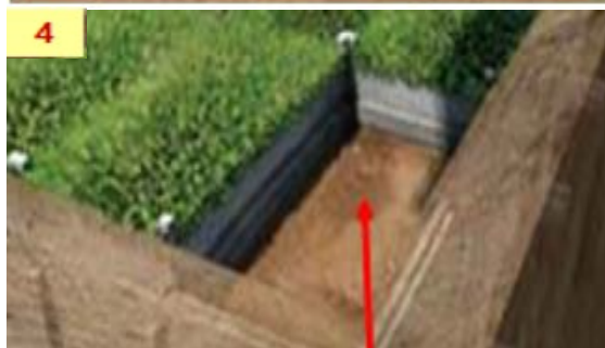
Backfilling of occupied CBS crypt
