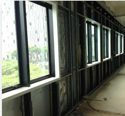
External interior walls are partition boards that have to be replaced
