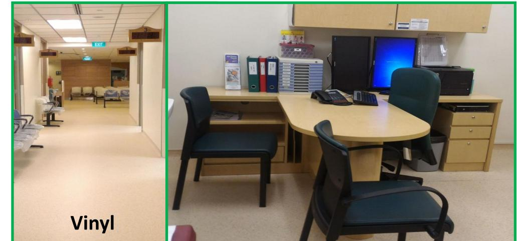
Carpeted flooring was replaced with vinyl flooring in adherence to infection control standards. With the new flooring, the floor can be more readily disinfected especially after spills of blood or other bodily fluids.
