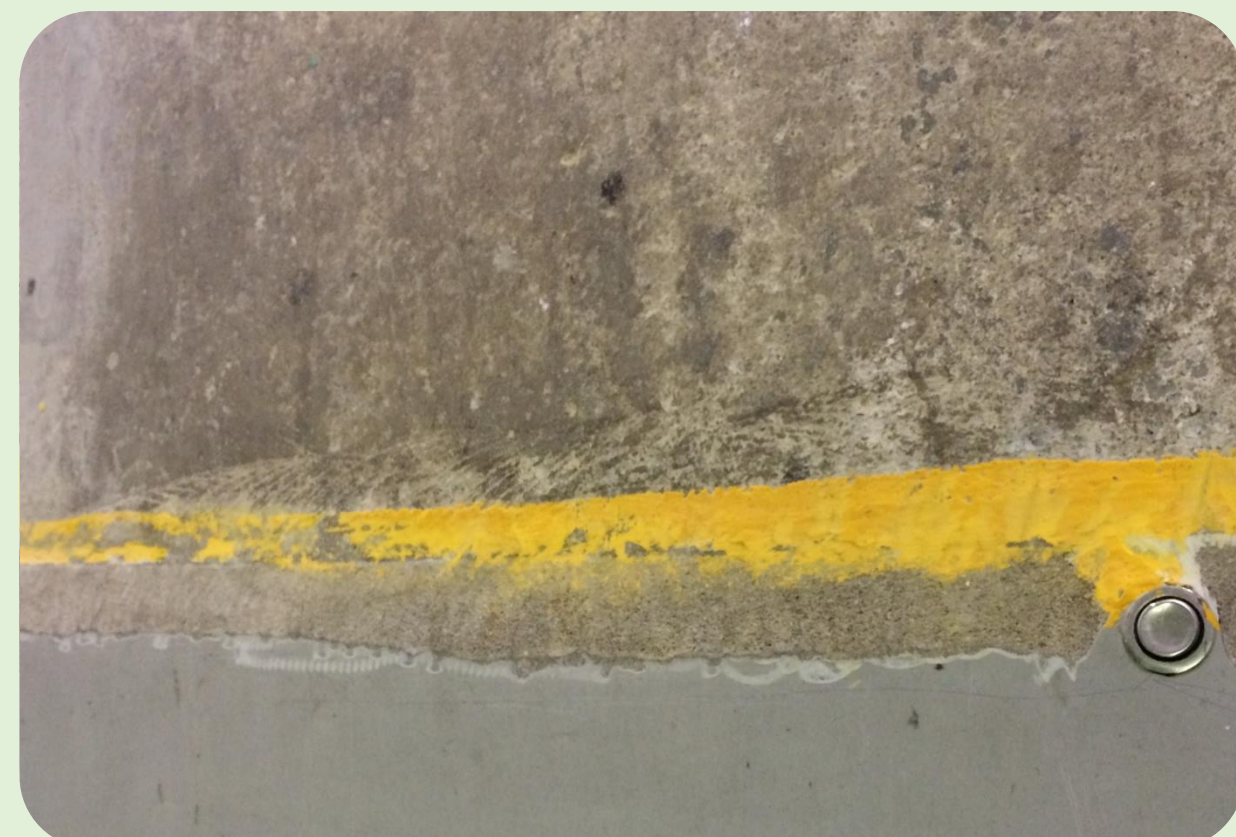
After: Damaged flooring repaired. Yellow lines drawn to mark elevated grounds.
