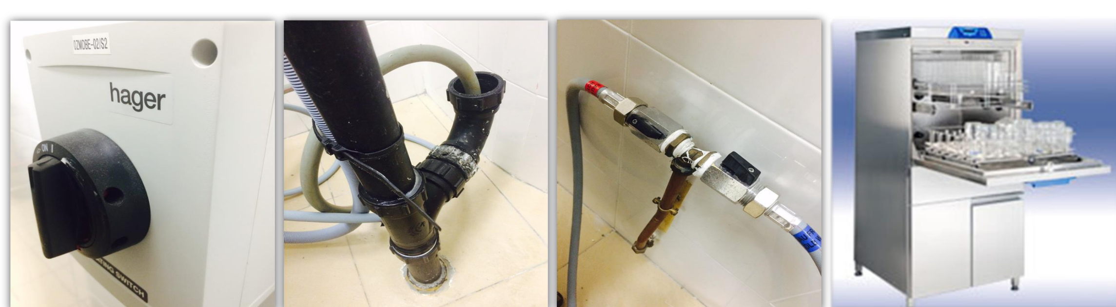
Figure 2 (left to right) : Hazards that were identified included need for a 13 Amp electrical socket, drainage pipes, water source and decommissioning, draining and disposal of existing unit.
