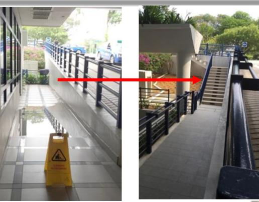
Built a direct, well-lit, anti-slip staircase linking street level and B1 to reduce the no. of slips and falls on the vehicular ramp
