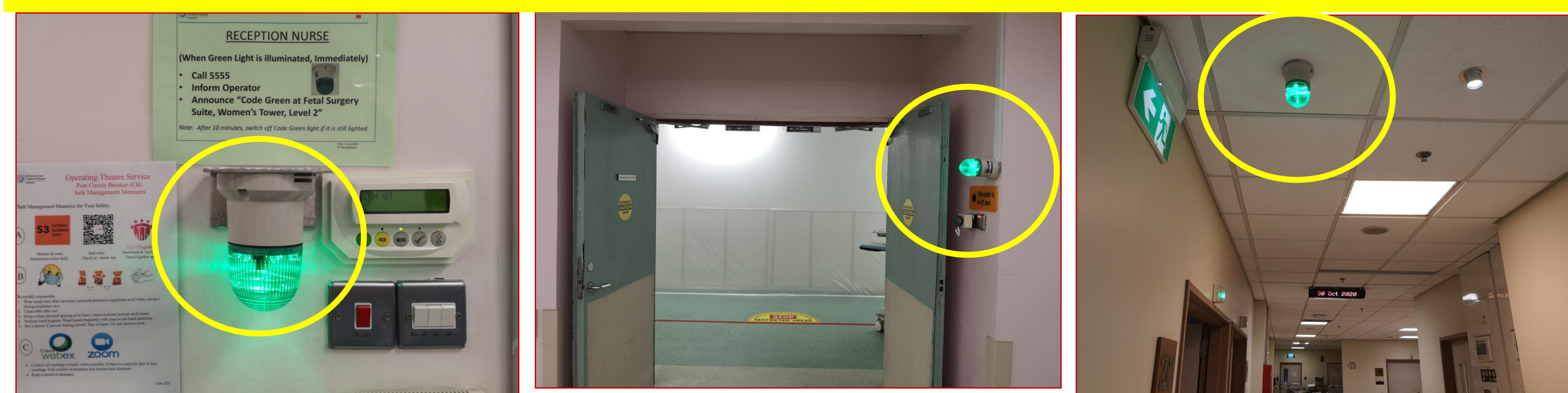
Women's OT Reception OT Emergency Door 2 Delivery Suite Corridor (ED 2)
