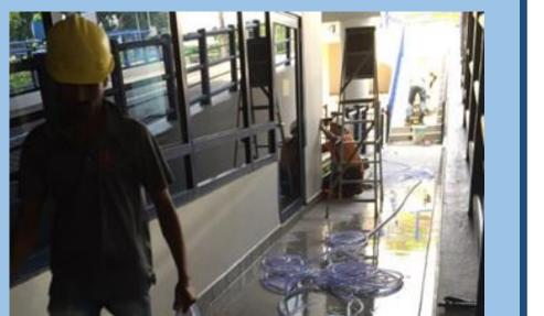
4c. Improved drainage along the footpath beside the ramp to eliminate potential slips & falls due to water-ponding. Resurfaced the footpath with anti-slip tiles to improve pedestrian safety during wet weather.
