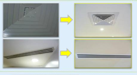
The project was able to eliminate water forming on the diffusers as a result of condensation. This in turn reduces the amount of reactionary effort needed to respond to the forming of water puddle on the ground. This design was made to promulgate to the other parts of the hospital.
