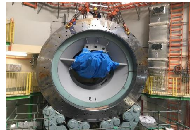
Installation of Gantry Parts
